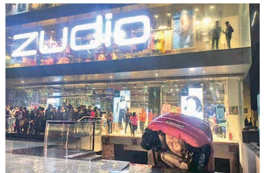
A driver lost control of his speeding car, causing the vehicle to crash into the basement of a Zudio showroom opposite Gaurav Tower in Jaipur on Sunday. No one was reported hurt in the incident.
